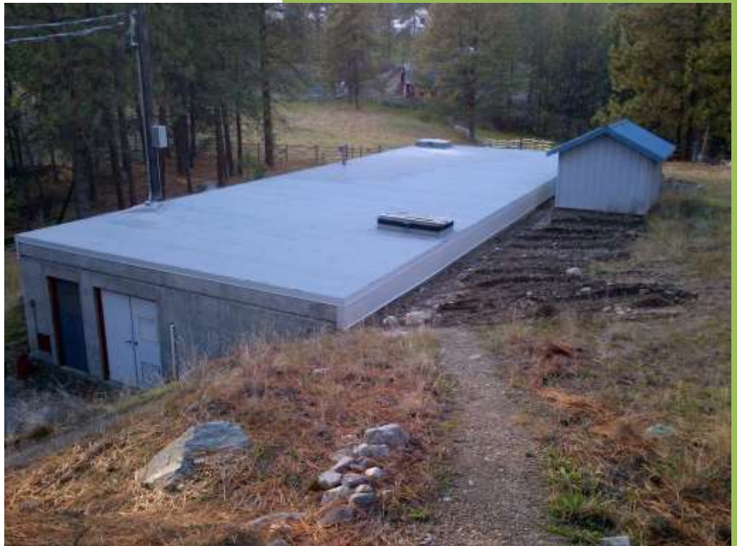
Sun Valley Pump Station and Reservoir
