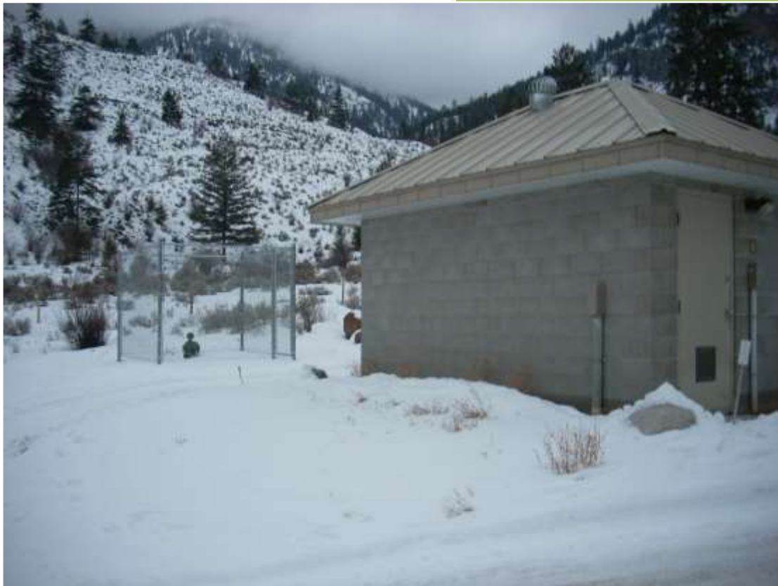
Olalla Well Pump Station
