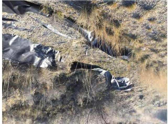
Photo 6 Ditch line maintenance measures in disrepair, on Sage Mesa Rd above WOW Golf Course
