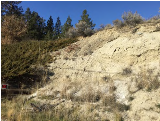
Photo 19 Colluvial silt and sand and gravel contact (end of Jonathan Dr.)
