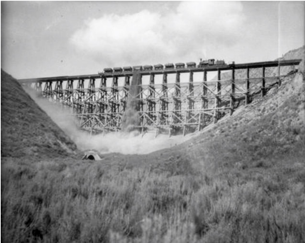
Figure 5.4.a Side dumping on KVR Trestle, at Mile 2.2 (Vancouver Archives: Item CVA 289-002.426, circa 1923) (likely located at the big gully north of Newton Drive)
