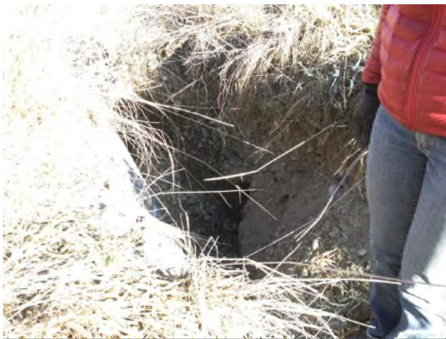
Photo 7 Erosion at Culvert Inlet at Sage Mesa Rd crossing (near WOW GC)
