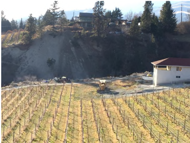
Photo 23 Fill dumping and shallow instability along gully slope (end of Moorpark Dr.)
