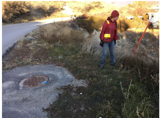
Photo 4 Catch basin above Sage Mesa Road at top of steep embankment (showing signs of instability)
