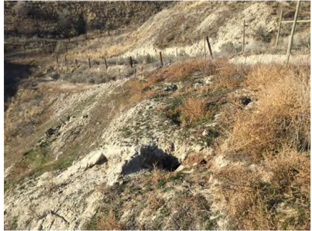
Photo 26 Sinkhole visible within gully (off Sparton Road)
