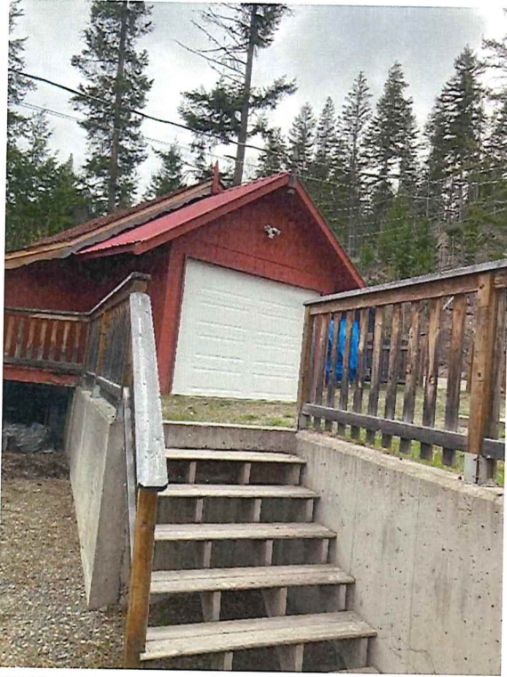
PHOTO 1: LOOKING SOUTHWEST AT WALKWAY INTO PROPERTY AND STORAGE GARAGE.
