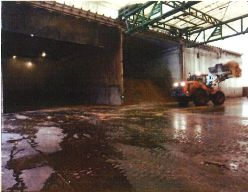
Enclosed Bunker System
