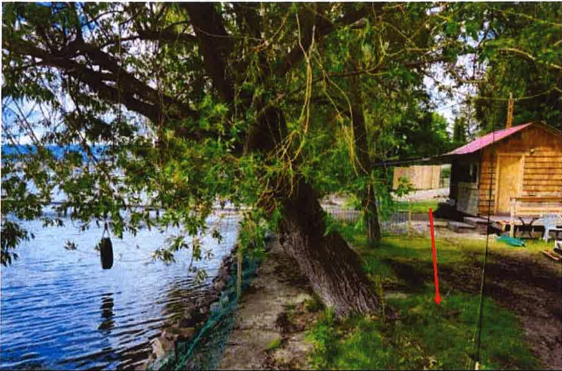
Pic 3 – June 11, 2022 – View looking at the Pacific Willow on 4535 Mill Rd. The root wad on the base of the tree on the right is lifting due in part to the tree lean; several large roots are exposed. This tree is in danger of falling over from the tree lean alone. A large stress fracture was also observed (see photo below).
