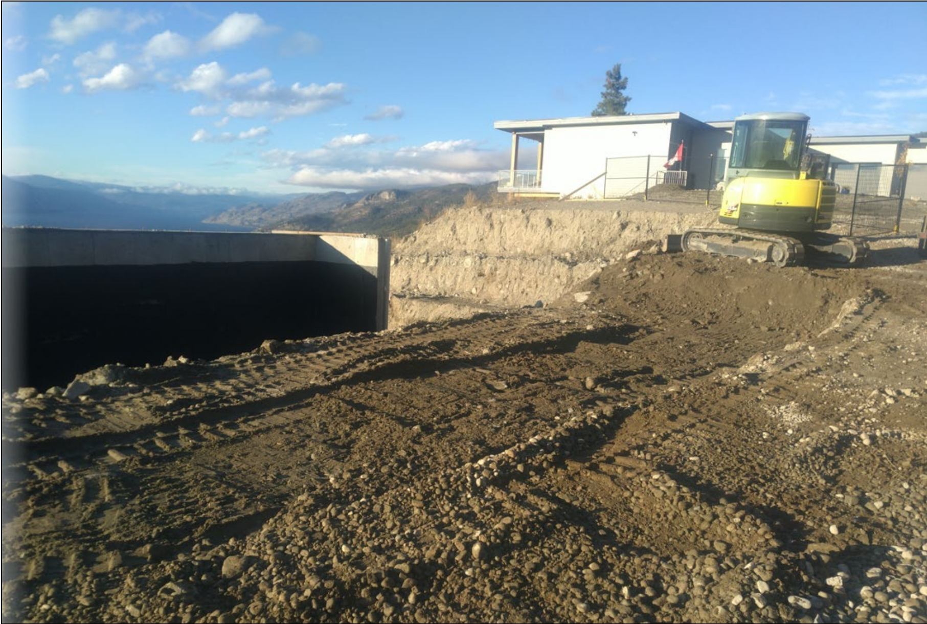
Attachment No. 3 – Site Photo facing northwest (November 2021)
