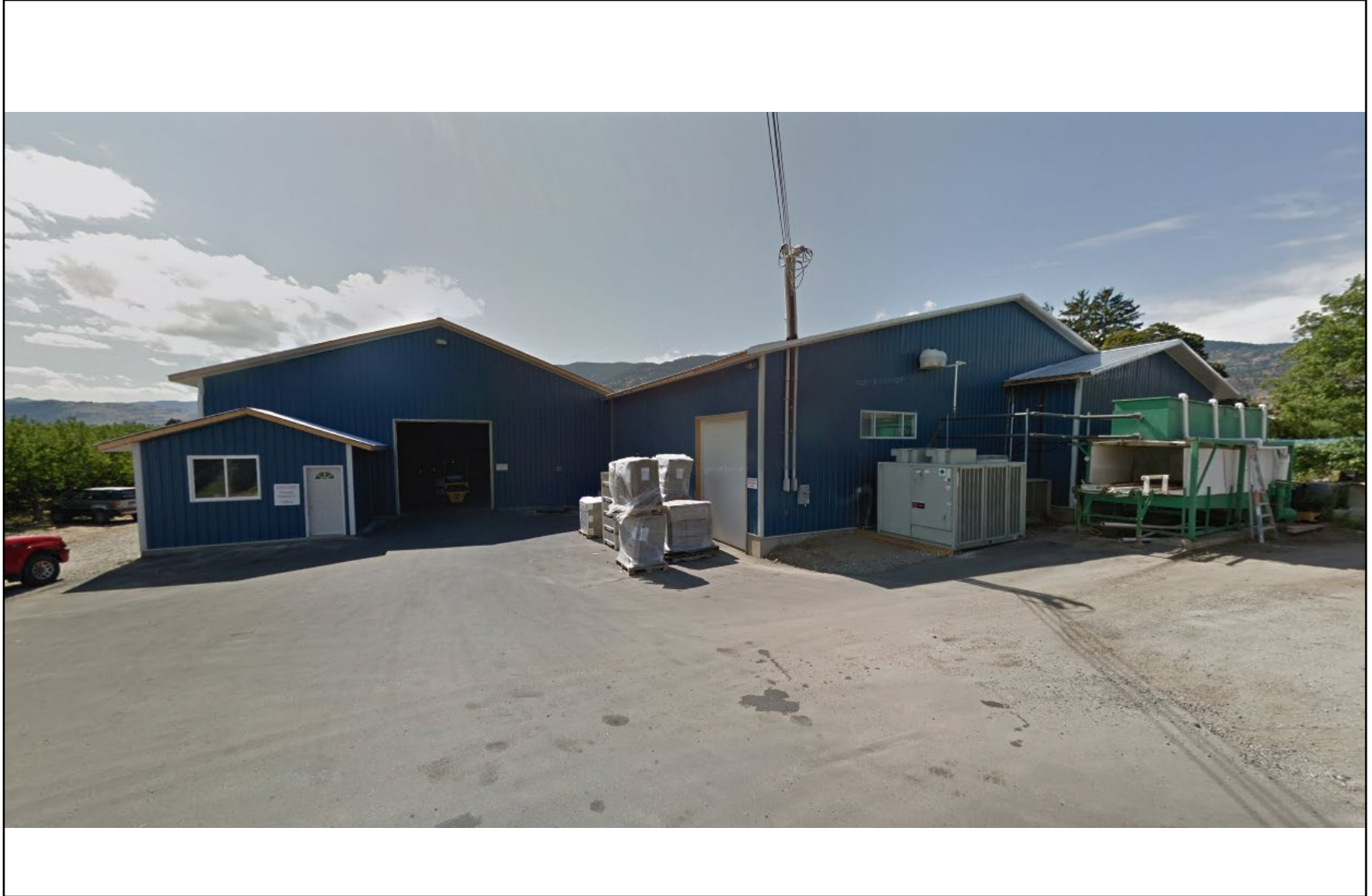
Attachment No. 3 – Site Photo; Existing Warehouse from Road 2 (Google Streetview – 2012)
