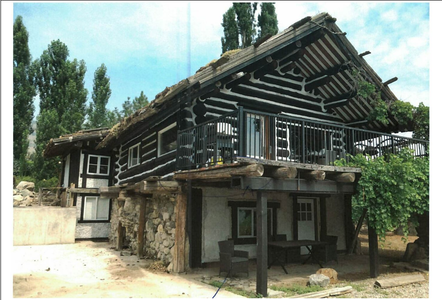
Attachment No. 4 – Site Photo (from health and safety inspection)
