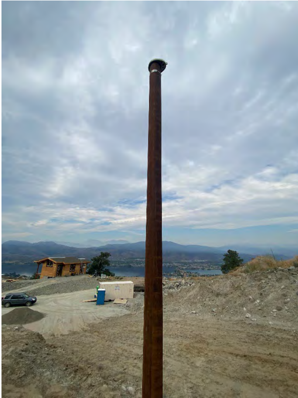
1. View of well casing stick-up on WTN 124408 (WPID 62040). Subsequently cut down to nominally 0.6m above current grade to facilitate test. View looking West.
