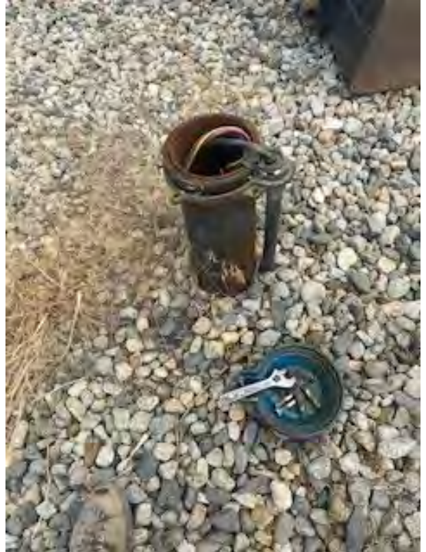
5. View of observation well WTN 84786, Driveway Well on neighbouring property to the west of site. Acoustic sounder used to monitor level. View looking southeast.
