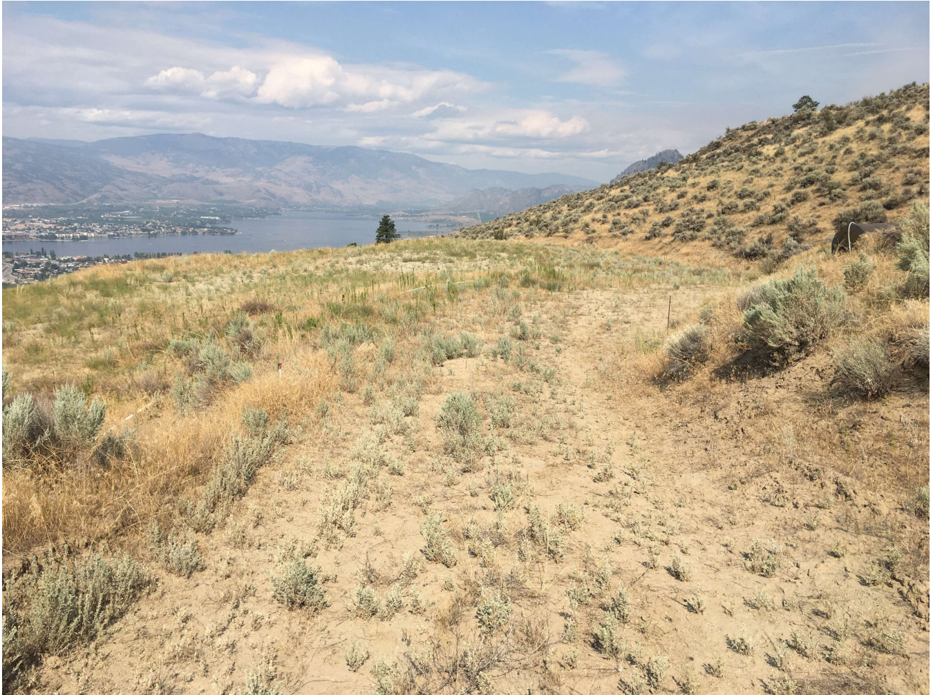
Photo 11 View of the uncontrolled fill area looking north prior to the stockpiling of blast rock in this area, photo looking north.
