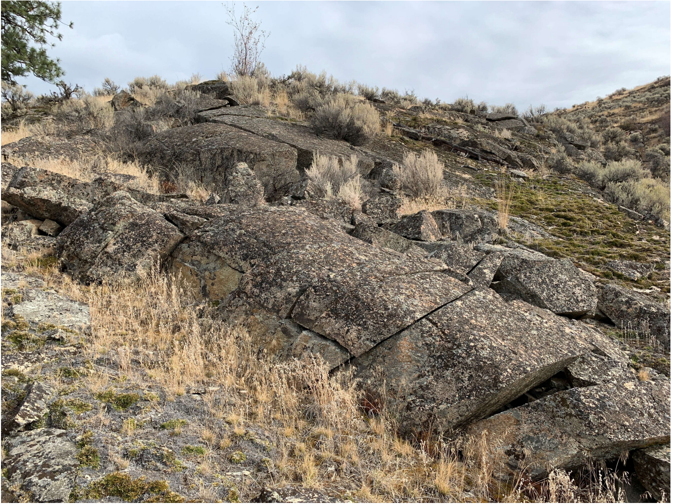
Photo 6 View of smooth bedrock outcrop east of access road with planar failures visible. Photo looking east.
