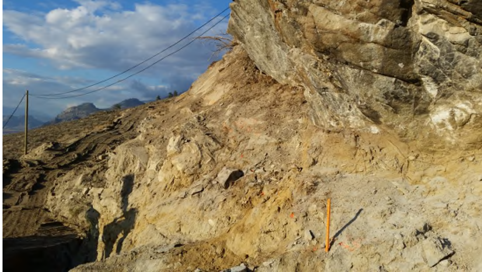
Photo 1 Rock slope exposed by blasting along the access road, November 20, 2015.
