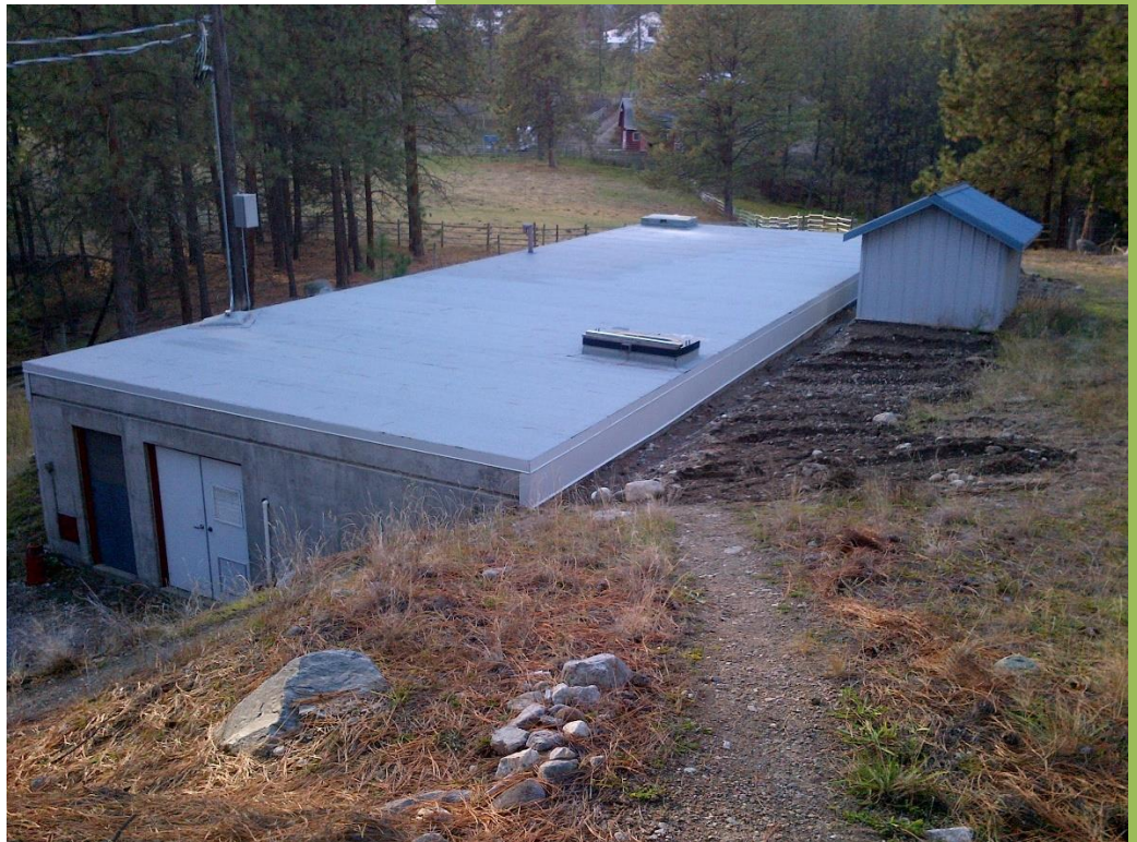
Sun Valley Pump Station and Reservoir
