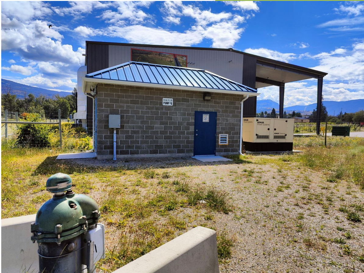
Okanagan Falls Well #6 Pump Station
