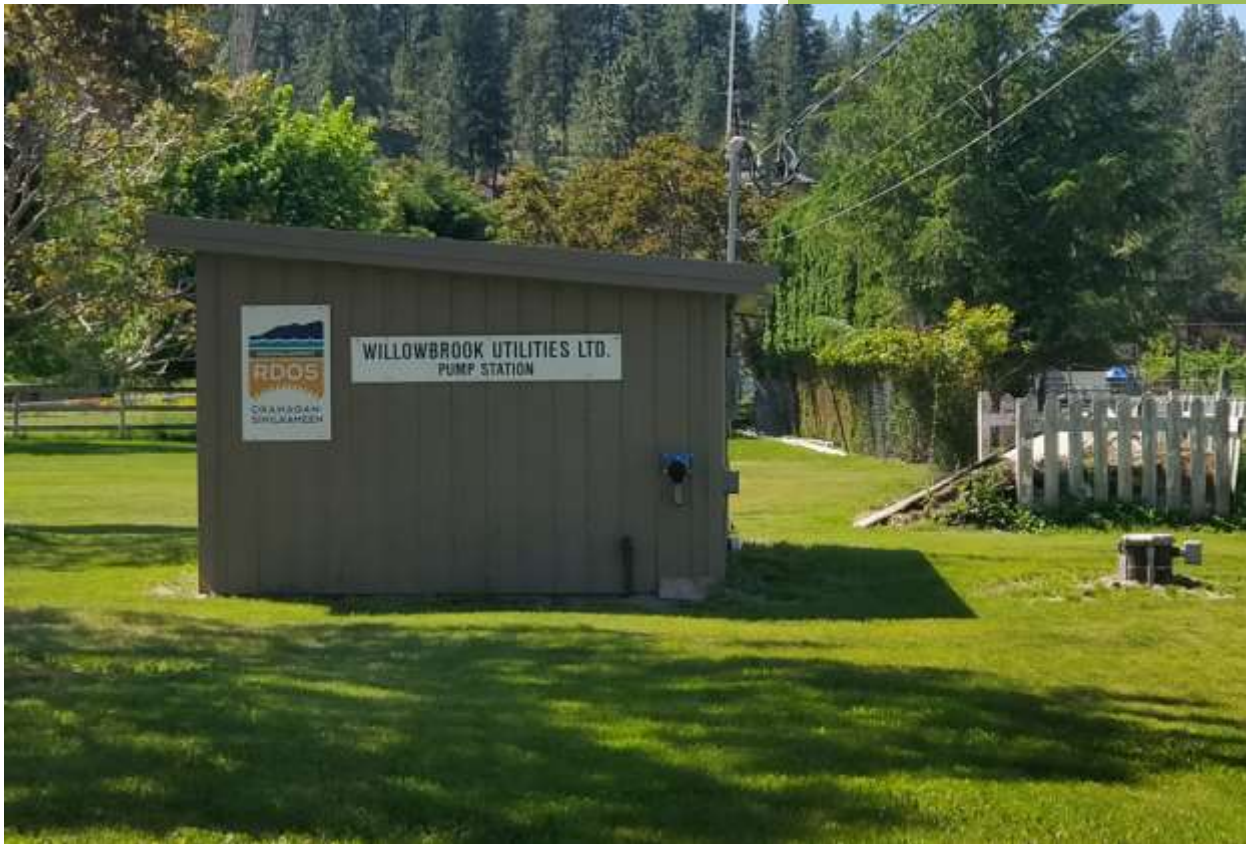
Willowbrook Well Pump Station
