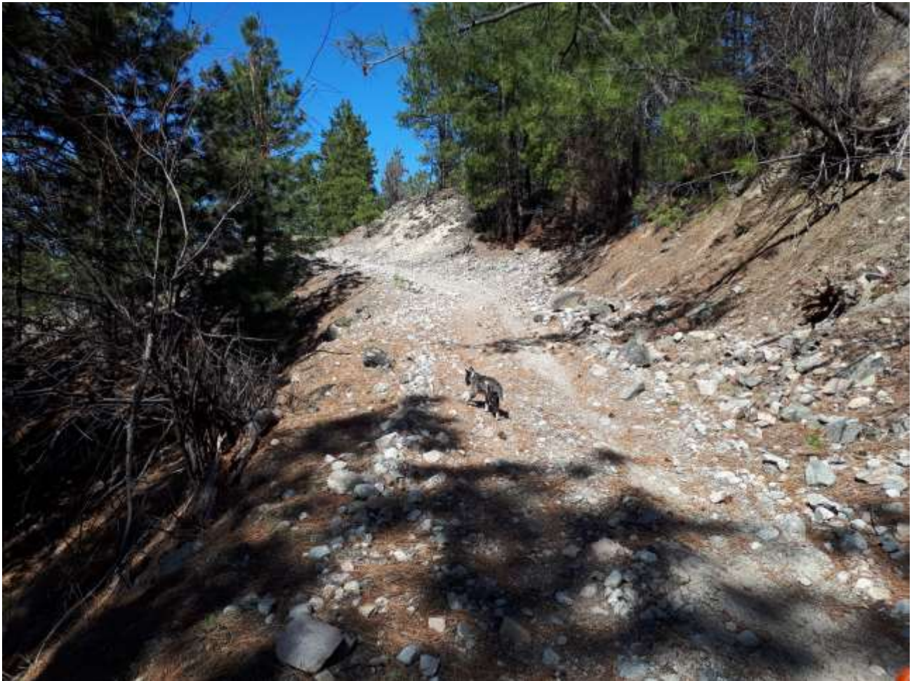
Photo 2: Looking north at existing access road entering the proposed subject property. Note the tills seen with road cut and spoil sluffing onto road.
