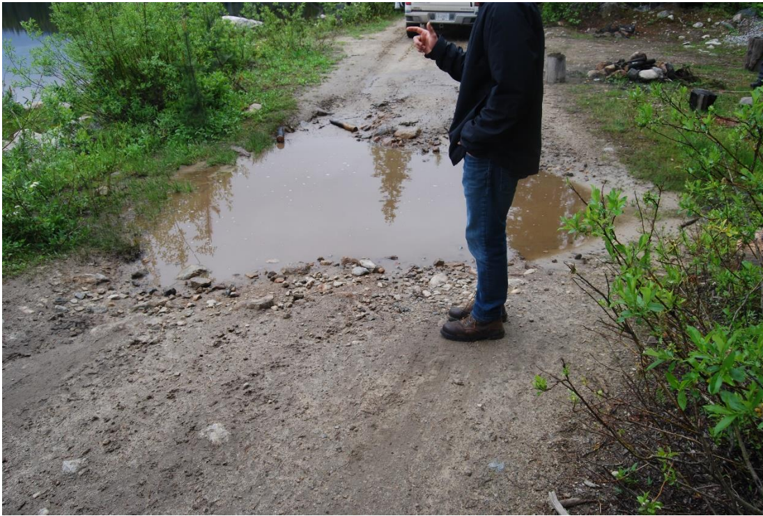
Photo A13: Big Meadow Lake Dam Low Crest Area close to Left Abutment
