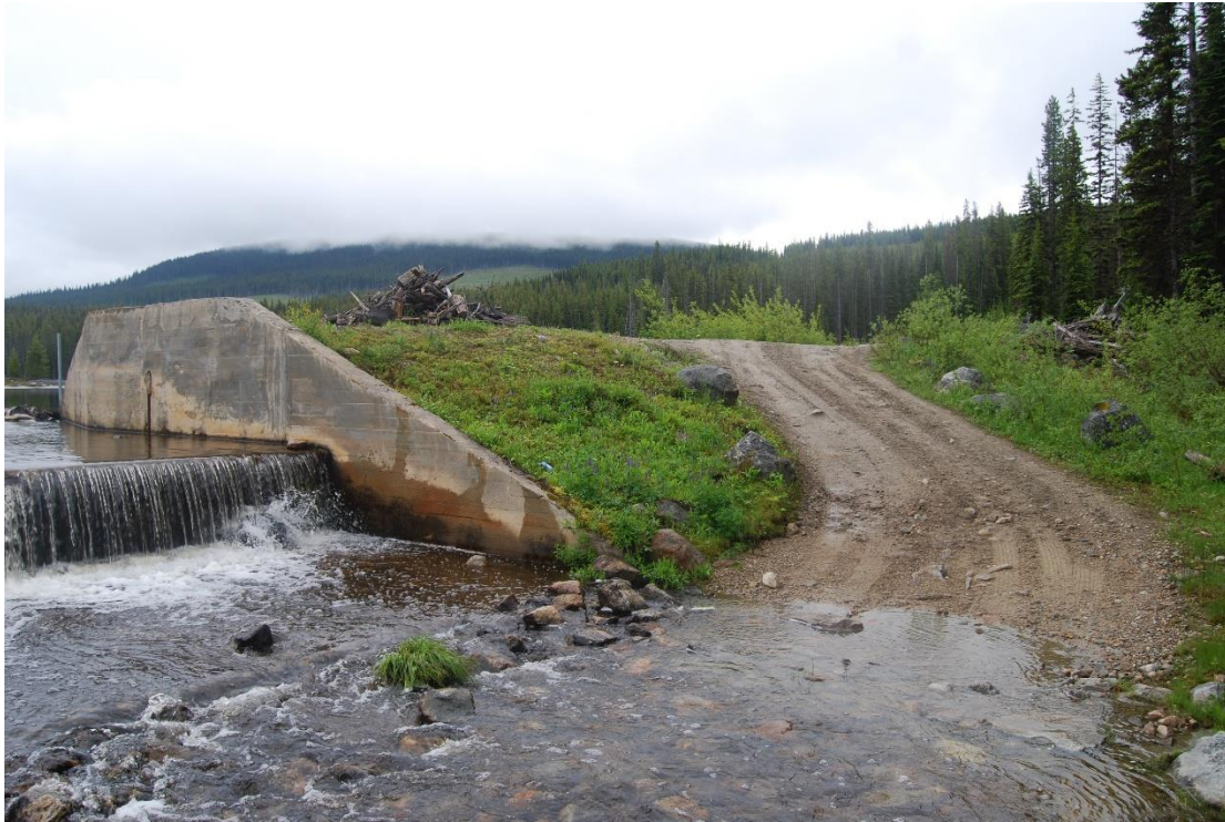
Photo A11: Big Meadow Lake Dam Spillway Downstream Channel and Access Road
