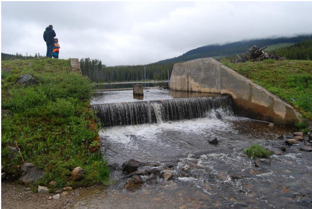
Photo A10: Big Meadow Lake Dam Spillway Structure
