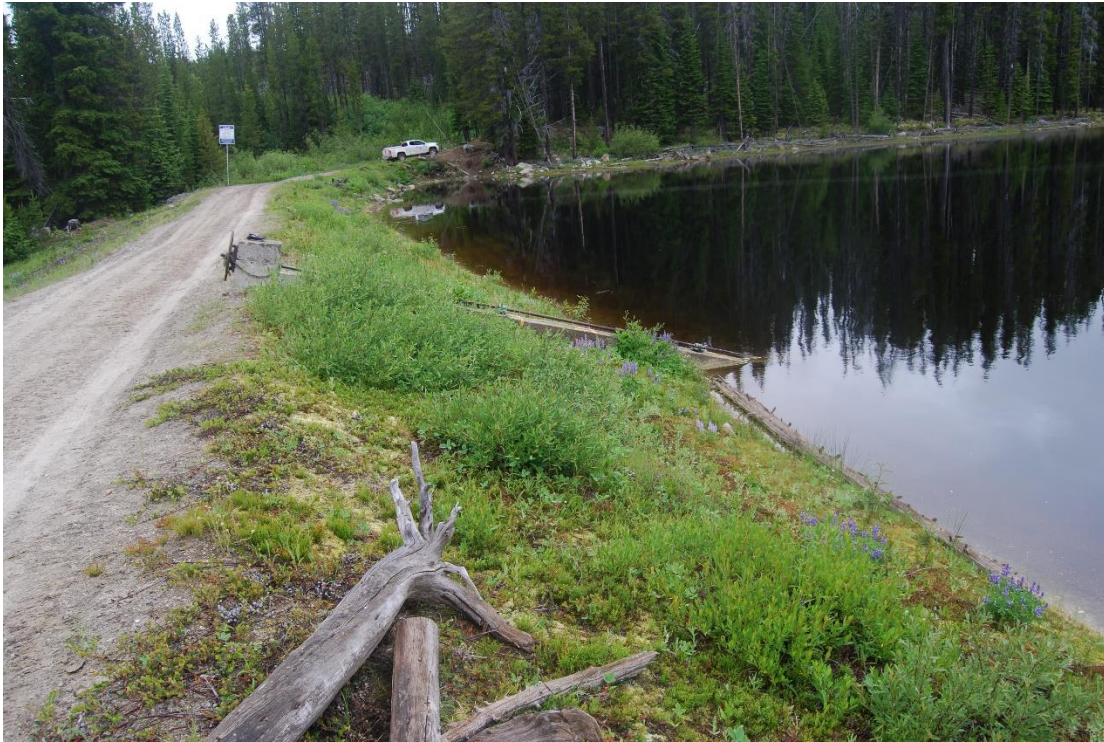
Photo A9: Big Meadow Lake Dam, Intake Structure and Dam Crest
