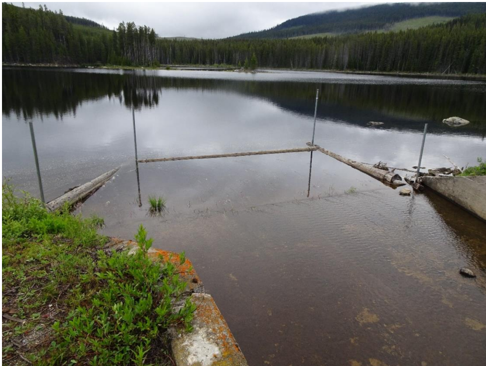
Photo A16: Big Meadow Lake Dam Debris Boom in Front of Spillway Structure
