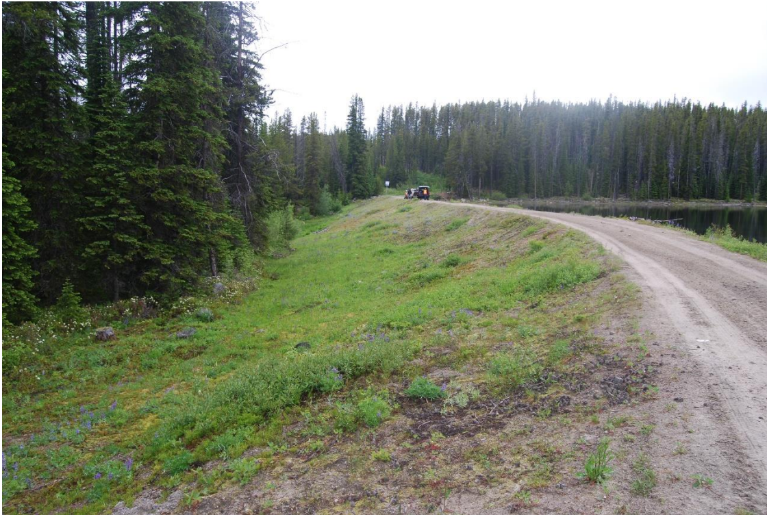
Photo A8: Big Meadow Lake Dam Downstream Slope and Dam Crest
