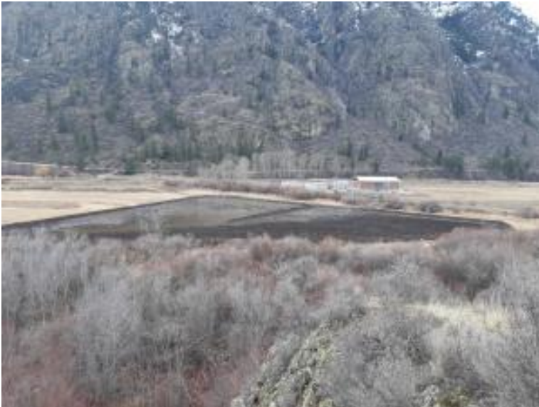
Current site of wetland under construction
