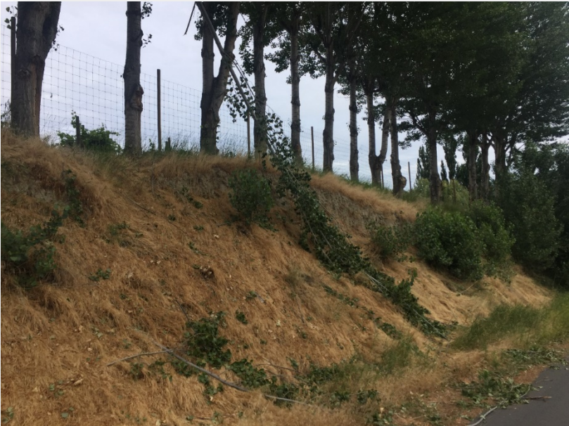
Figure 20 Shoulder vegetation along Spruce Avenue, a summer maintenance class 6 road, and as such not included for shoulder mowing in the current highway maintenance standards.
