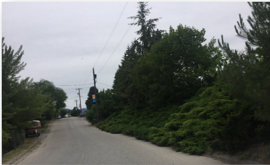
Figure 19 Looking south on Linden Avenue. This road is summer maintenance class 5, which is included for shoulder mowing in the current highway maintenance standards. This photo depicts an extensive clump of juniper that have spilled onto the road from an adjacent property.
