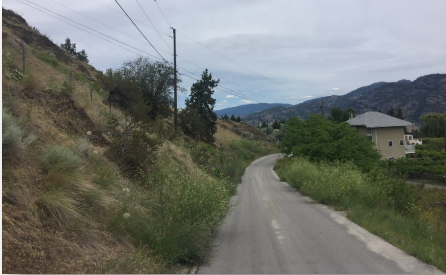
Figure 18 Looking north east down Dogwood Avenue. This road is summer maintenance class 6, which is not included for shoulder mowing in the highway maintenance standards that are currently in effect.
