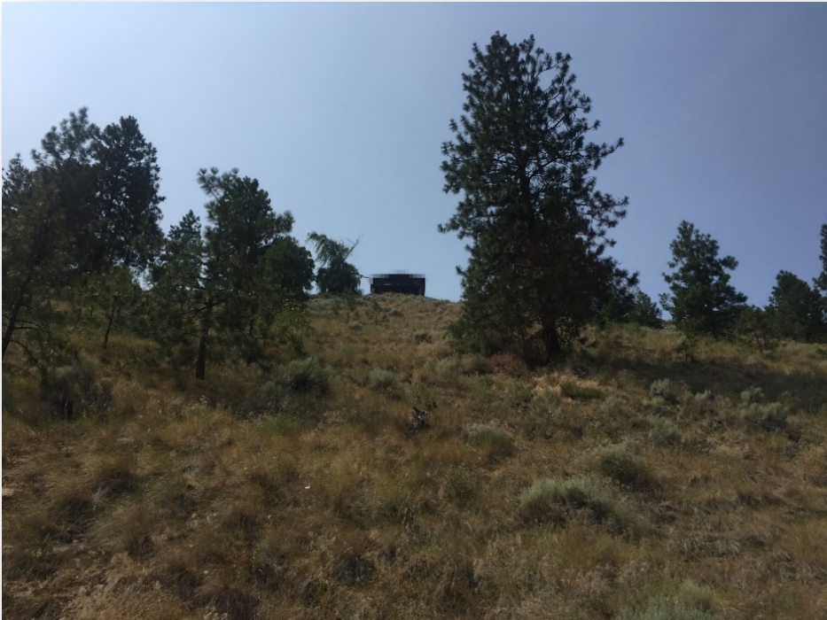
Figure 27 No set back between the home and a 70% slope below. In addition, an overhanging deck and home further exposes the home to upslope fire spread and direct flame contact.
