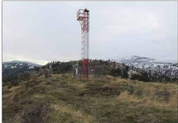
Picture 1: Kaleden E911 Radio Communications Site
