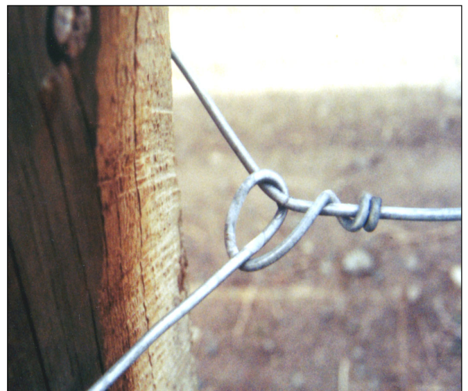
Figure 6 Tying Off Woven Wire (top view)
