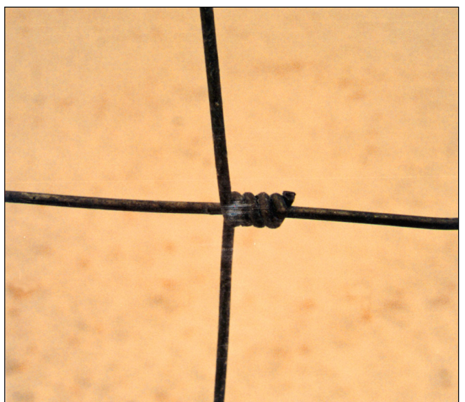
Figure 2 Hinged Joint
