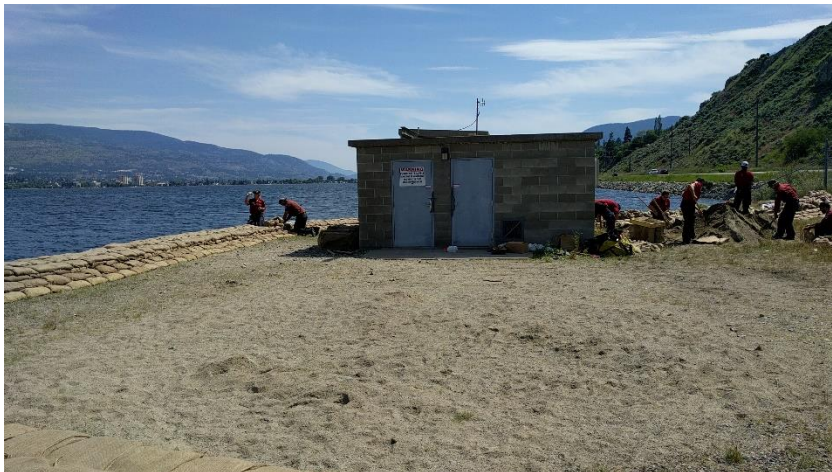
Photo 8: Sandbagging intake pump house during 2017 flood
