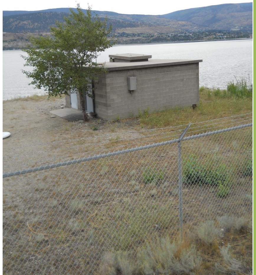
Sage Mesa Lake Pump Station
