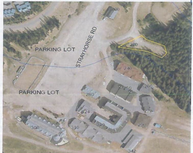
Lease area shown in top right (yellow outline). Area used currently for overflow parking and waste bins.
