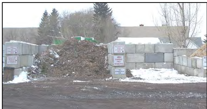
Exhibit 5- 3: Typical bunker-style depot constructed from ecology-blocks.
