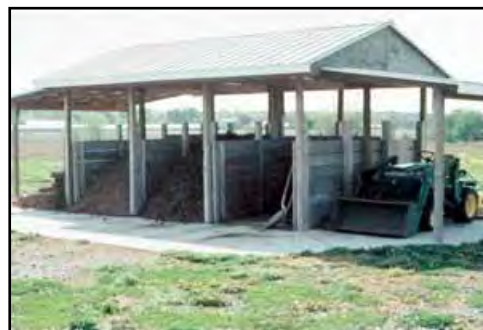
Exhibit 6- 3: Small bunker composting system used to process animal manures.
