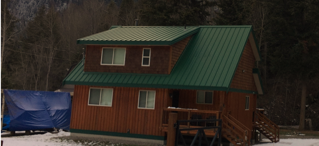
Figure 7 Roofs with a ULC rating, such as this metal roof, provide a high degree of fire resistance able to withstand ember ignition.
