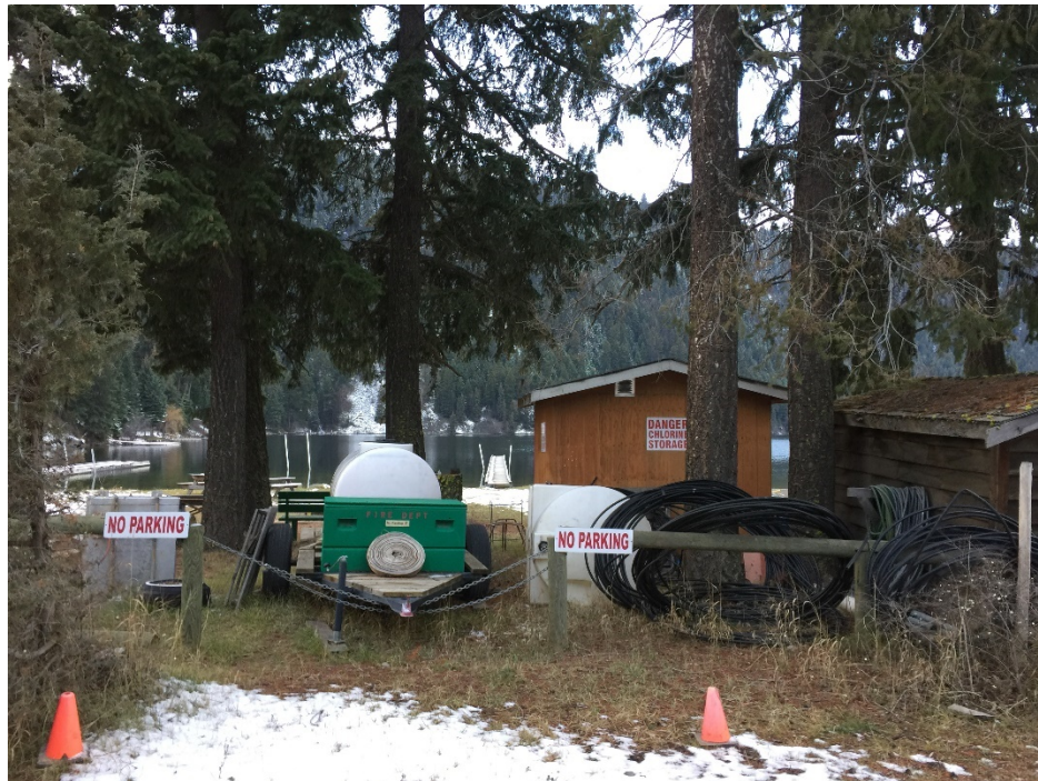
Figure 14 Missezula Lake owners have several portable water tanks and various firefighting equipment staged at the water treatment plant.
