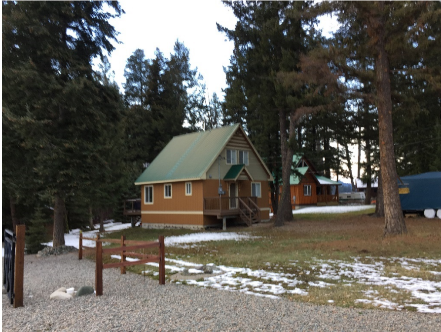
Figure 11 Steep-pitched metal roofs are common at Missezula Lake. This property is also a good example of a fuel-managed Zone 1 with occasional well-pruned and spaced large diameter conifers.
