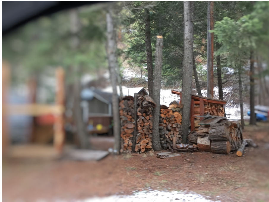
Figure 8 The presence of nearby vegetation and combustibles that can ignite with relative ease and burn with high-intensity can present a fuel hazard to a building's exterior.
