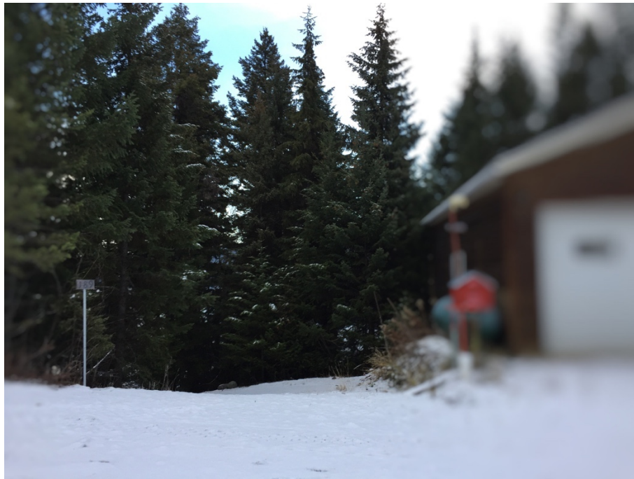
Figure 9 The conifer trees in this photograph have ladder fuels extending down to the ground. This is an example of Zone 1 conifers presenting a hazard to the adjacent structure.
