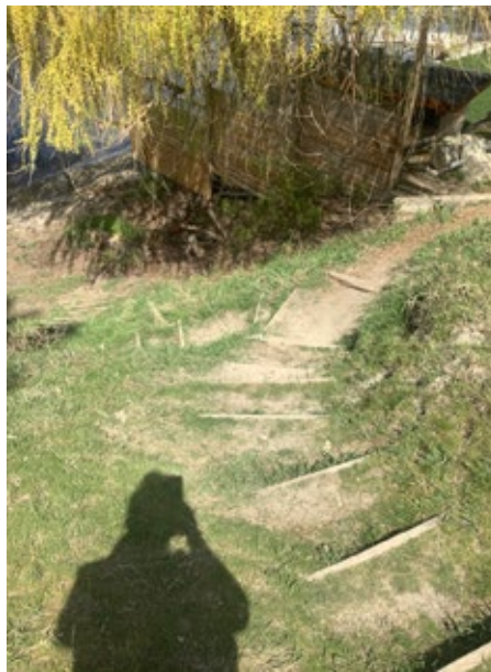
Failing & Inaccessible Stairs Leading to the Water
